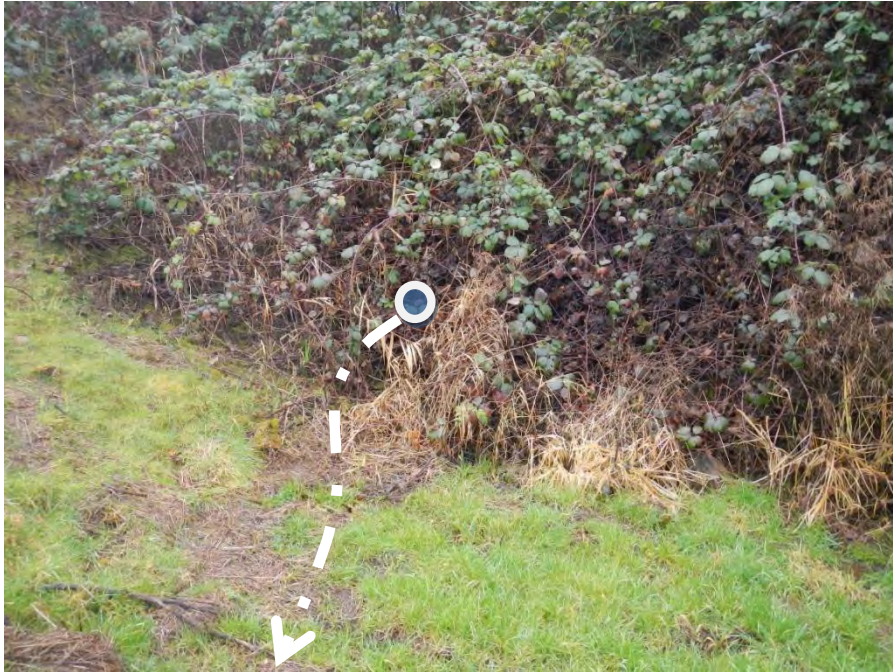
Figure 3.3.3 Looking south at 12" Culvert under existing driveway
