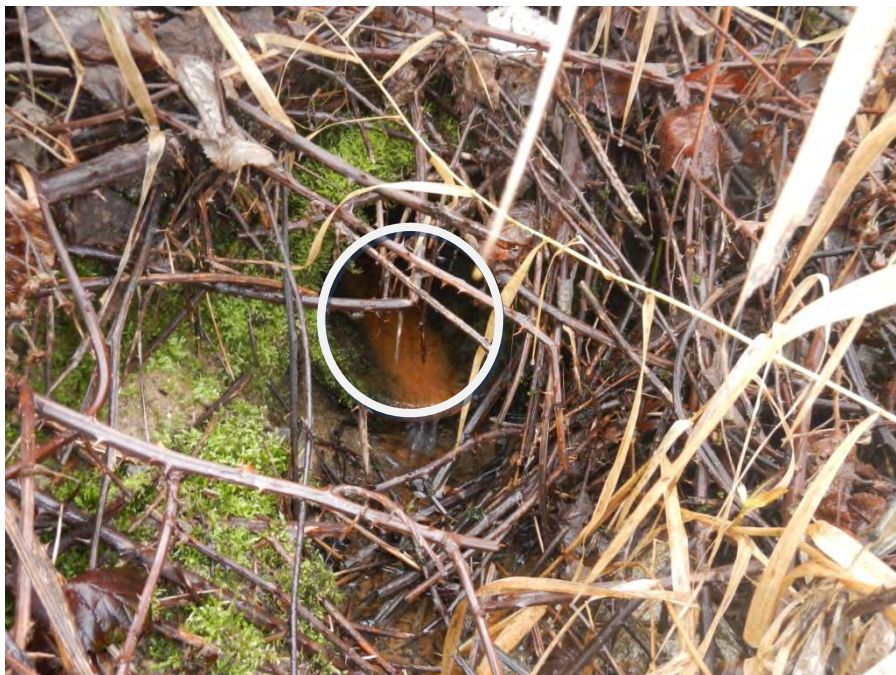
Figure 3.3.4 Close up of existing 12" Culvert
