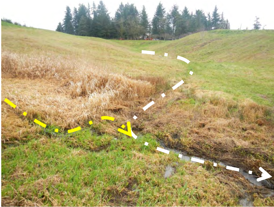
Figure 3.3.6 Continuation of Grassy Channel (Looking south 290° of Reach 2)
